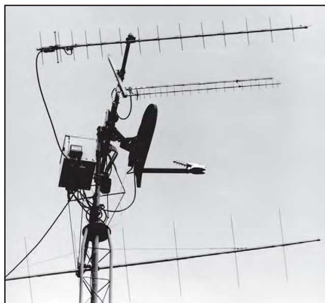
Fig 23.37 —Details of WD4FAB’s tower cluster of satellite antennas, including a home-brew elevation rotator. Top to bottom: M 2 436-CP30, a CP U-band antenna; two each M 2 23CM22EZA antennas shown in a CP array for L band; “FABStar” dish antenna with helix feed for S band; M 2 2M-CP22, a CP V-band antenna (only partially shown.) To left of dish antenna is a NEMA4 equipment box with an internal 40W L-band amplifier, and also hosts externally-mounted preamplifiers.
